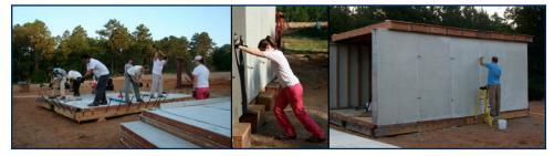
Ease of Assembly: A 12'x20' blast-resistant modular structure for force protection may be easily installed. After the foundation is level, the structure takes 90 minutes for 12 personnel to install.
