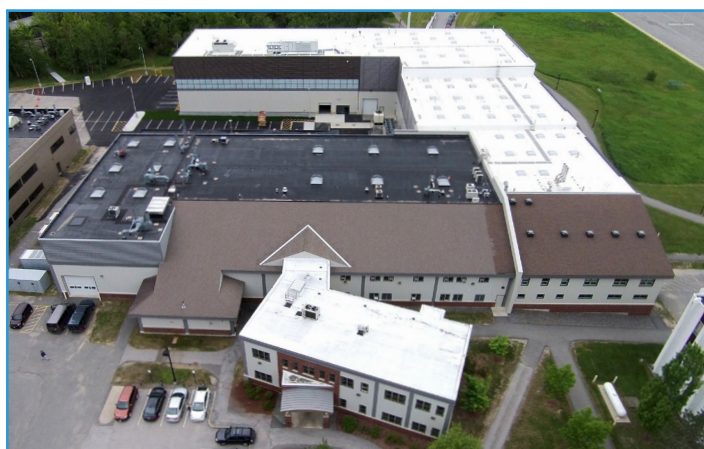
UMaine's Advanced Structures and Composites Center ISO 17025-accredited testing laboratory in Orono, Maine.
