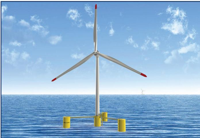
UMaine's patented VoltturnUS floating concrete hull technology that can support wind turbines in water depths of 150 feet or more, and has the potential to significantly reduce the cost of offshore wind.
